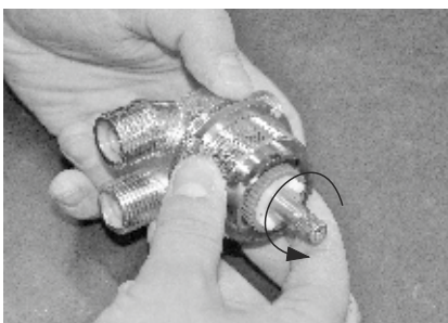
8. Unscrewing of the shower mixer head
