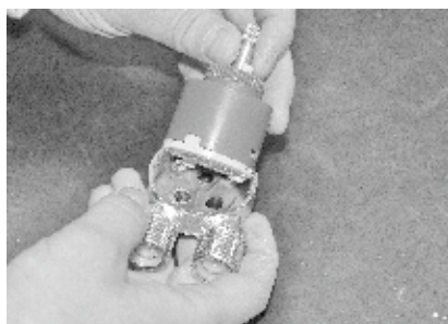
9. Pulling out the shower mixer head
