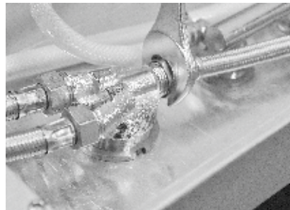
6. Detaching the water supply
